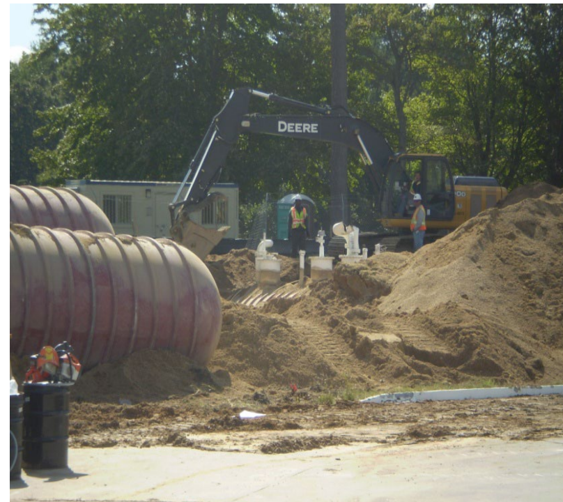
D-37 Aviation Fuel Tank Farm tanks removed to prevent groundwater contamination.
