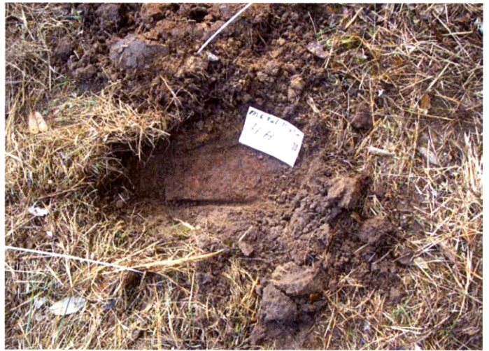
Surface Clearance – Steel Plate – Left in place Grid 4A
