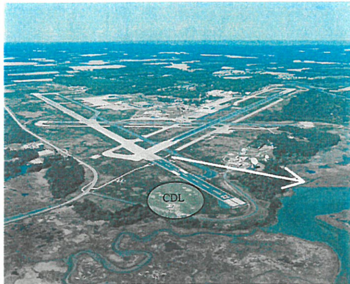
WFF: Former Construction Debris Landfill Area with North arrow (white)
