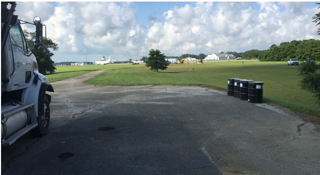
Photograph 53: Standing next to Building A-131 looking down the undamaged portion of the asphalt road. The IDW from the site was temporarily stored on the asphalt pad before being transported to Building B-29 by NASA personnel.
