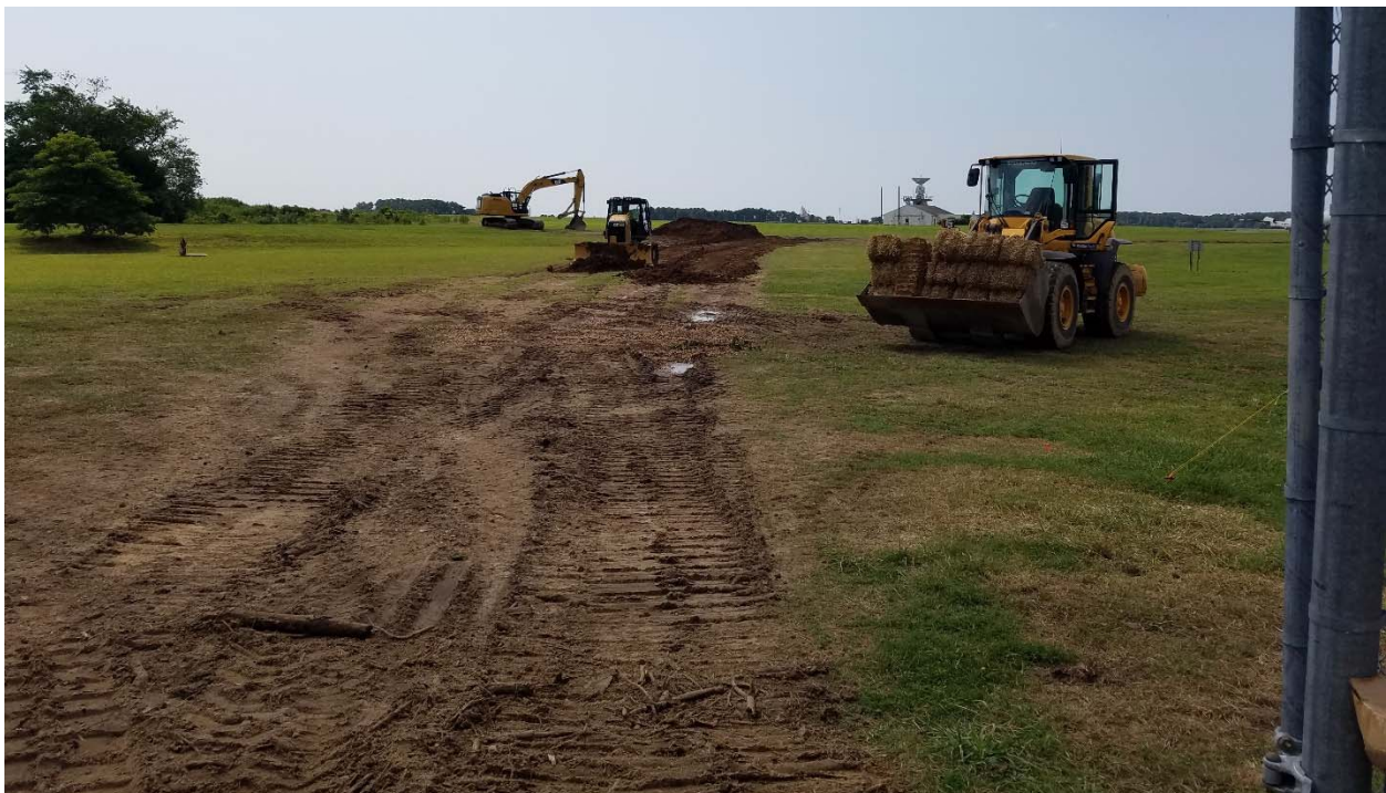
Photograph 47: Standing at the gate to the Pistol Range looking southeast at the access road during restoration activities. The soil stockpiled from the asphalt road repair was used to backfill the ruts.
