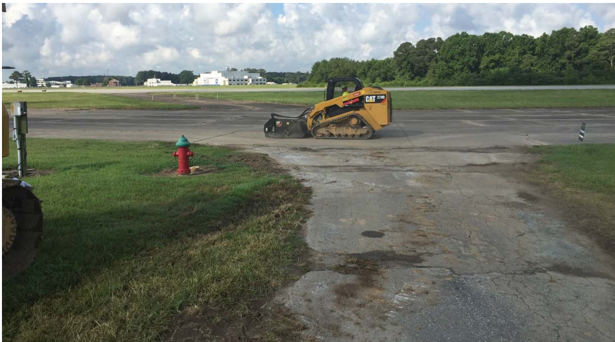
Photograph 57: Throughout the project, the roads adjacent to the airfield were swept to prevent road debris from making it out onto the runways.
