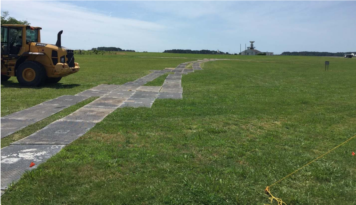
Photograph 44: Standing at the gate to the Pistol Range looking southeast at the access road. Traction mats were used to limit the effects of truck traffic on the landscape.
