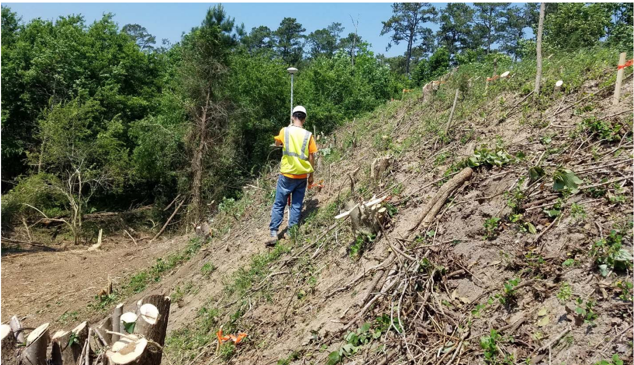
Photograph 29: Looking west across the Rifle Range target mound during the layout of the sampling/excavation grid. A GPS unit with an external antennae was used to locate grid corners.
