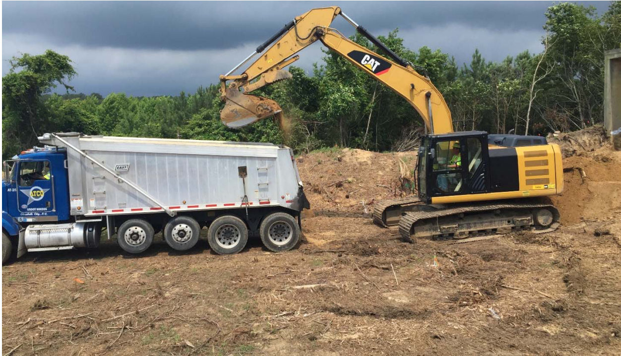
Photograph 11: Looking west at a truck being loaded with lead-impacted soil at the Pistol Range.
