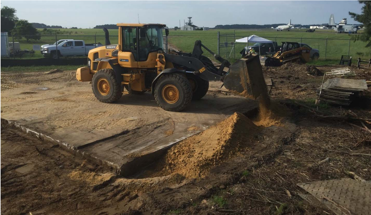
Photograph 19: Looking southeast at the backfilling of grids A3 and B3 at the Pistol Range.
