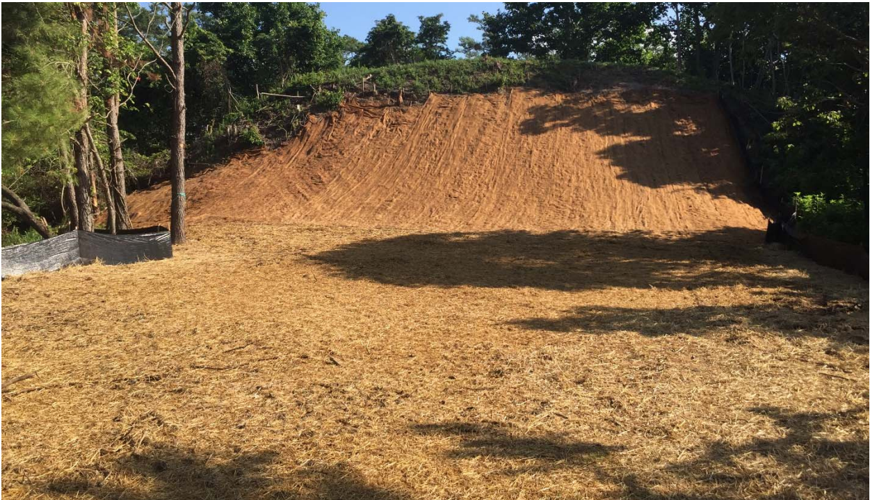
Photograph 43: Looking north at the Rifle Range target mound and flat portions of the site after seeding, fertilizing, and erosion control measures were completed.
