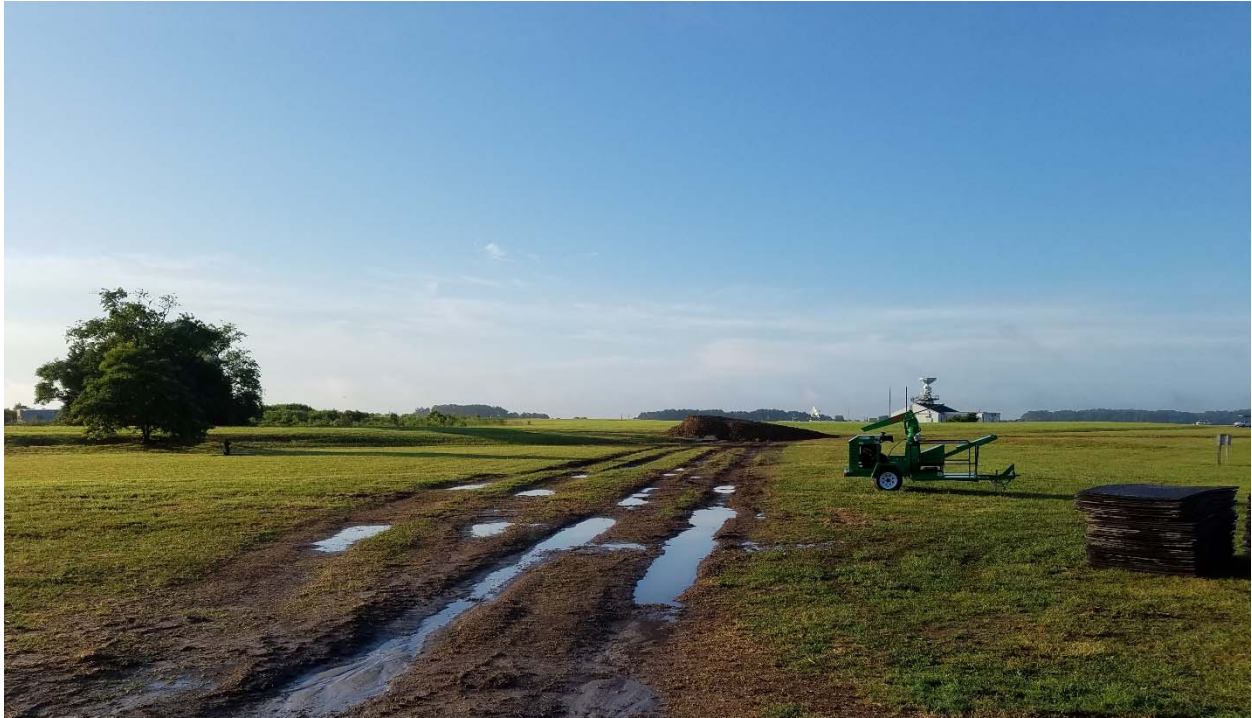
Photograph 46: Standing at the gate to the Pistol Range looking southeast at the access road after all truck traffic had passed. Note a heavy rainfall of approximately 2 inches fell the night before.
