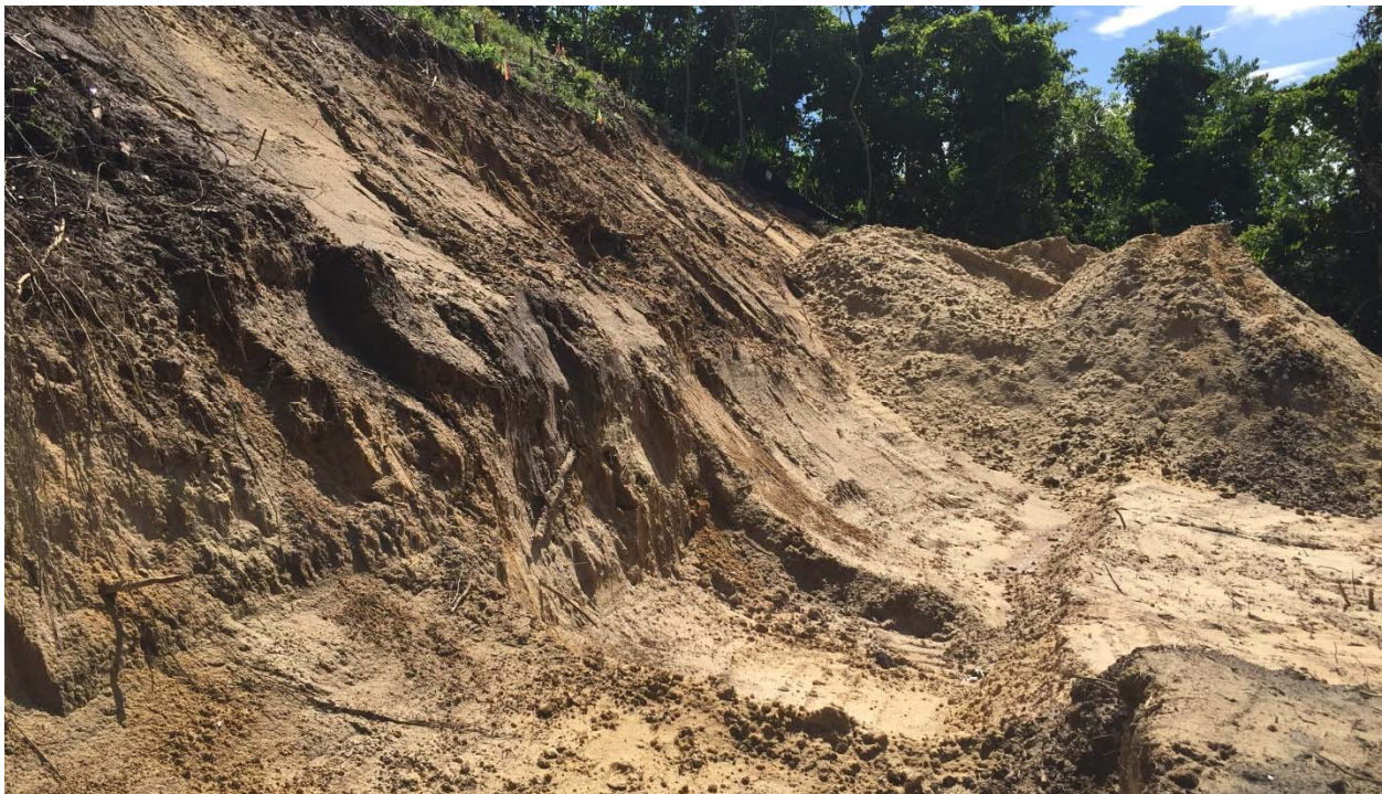
Photograph 35: Looking east across the Rifle Range target mound after all grids were dug out. The lead-impacted soil was stockpiled in grids C5, C6, B5, and B6 awaiting loading into trucks.
