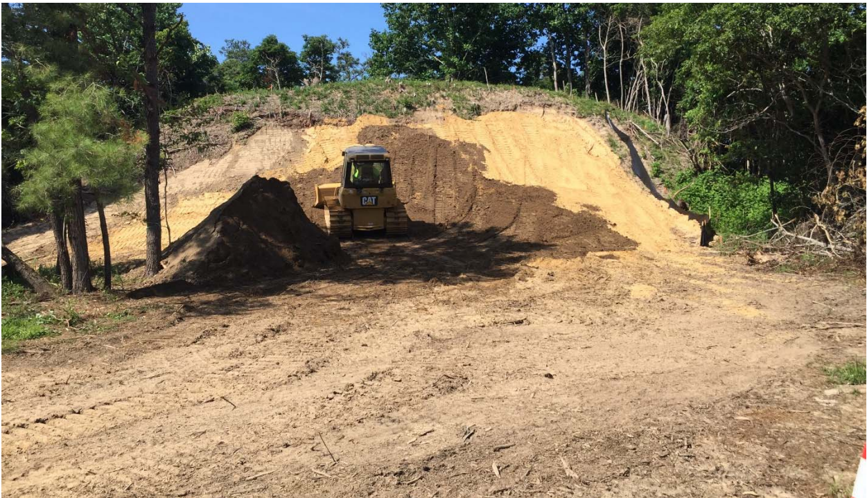
Photograph 39: Looking north at the Rifle Range target mound as top soil is being spread.
