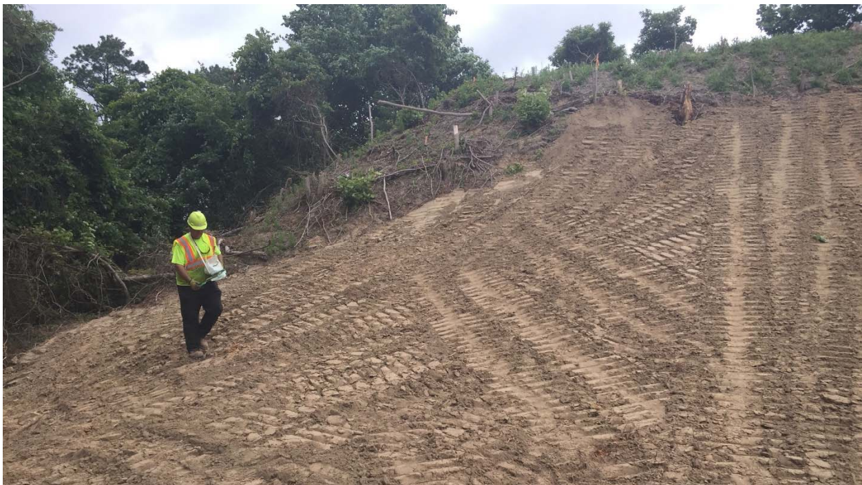
Photograph 41: A bag spreader was used to spread the seed at the Rifle Range target mound.
