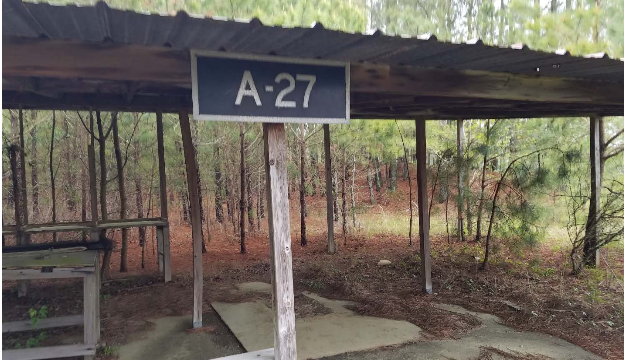
Photograph 1: Standing just south of the firing line structure, A-27, looking northeast towards the Pistol Range target mound. However trees are obscuring the view of the target mound.
