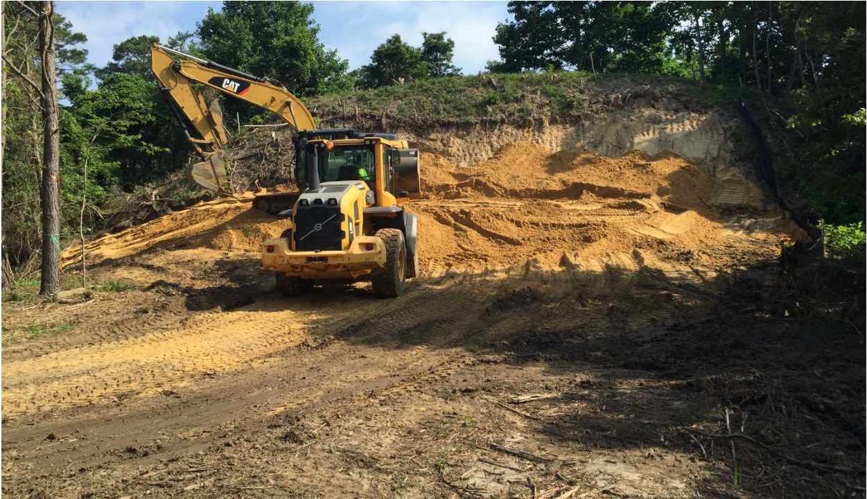
Photograph 38: Looking north at the Rifle Range target mound during backfilling.
