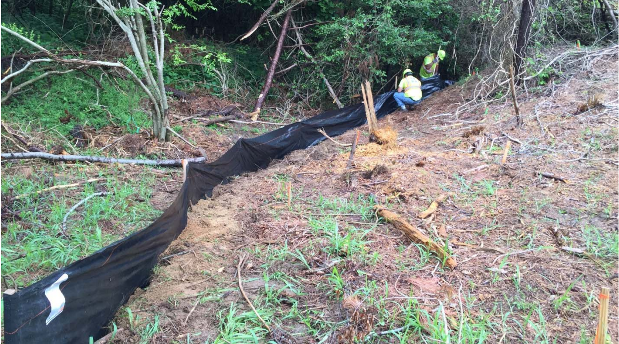
Photograph 32: Looking northwest at silt fence installation at the Rifle Range.
