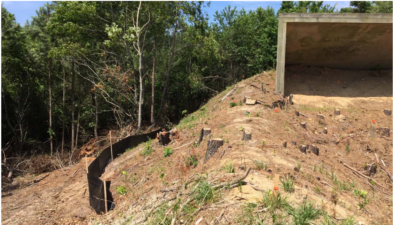
Photograph 6: Standing on the southern berm of the Pistol Range looking northeast at the silt fencing and target mound. Wood stakes indicate grid corners and pin flags indicate sampling locations.
