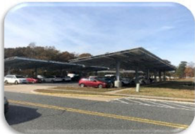
Solar Covered Parking
