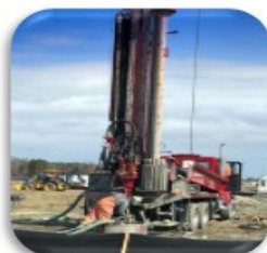
Geothermal Well Drilling for Heat Recovery Chillers
