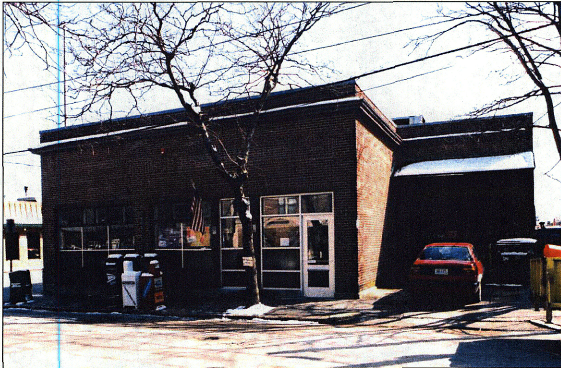
Figure 10 - North Elevation, 201 Meeting Street
