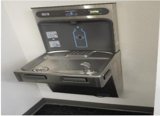
Greenbelt B33 Water Bottle Fill Station reduces waste of single use plastic water bottles
