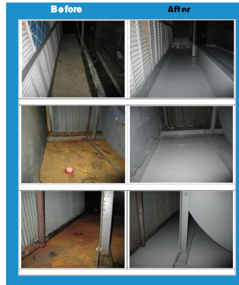
GB EBCx (ACS Refurbishment and Coil Restoration)
