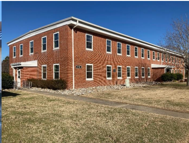
Building F-6 WFF Headquarters – GP Certified
