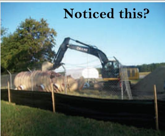
Aging underground storage tanks were recently excavated from the D-37 Aviation Fuel Tank Farm, removing a potential source of environmental contamination.
