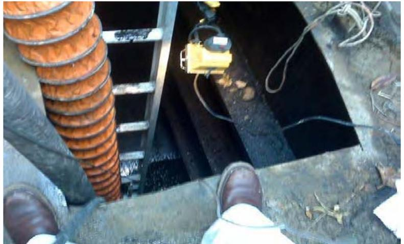
*Ventilation hoses provide air and exhaust toxic vapors during confined space entry. A guardrail would also be necessary to protect workers from potential falls.*
