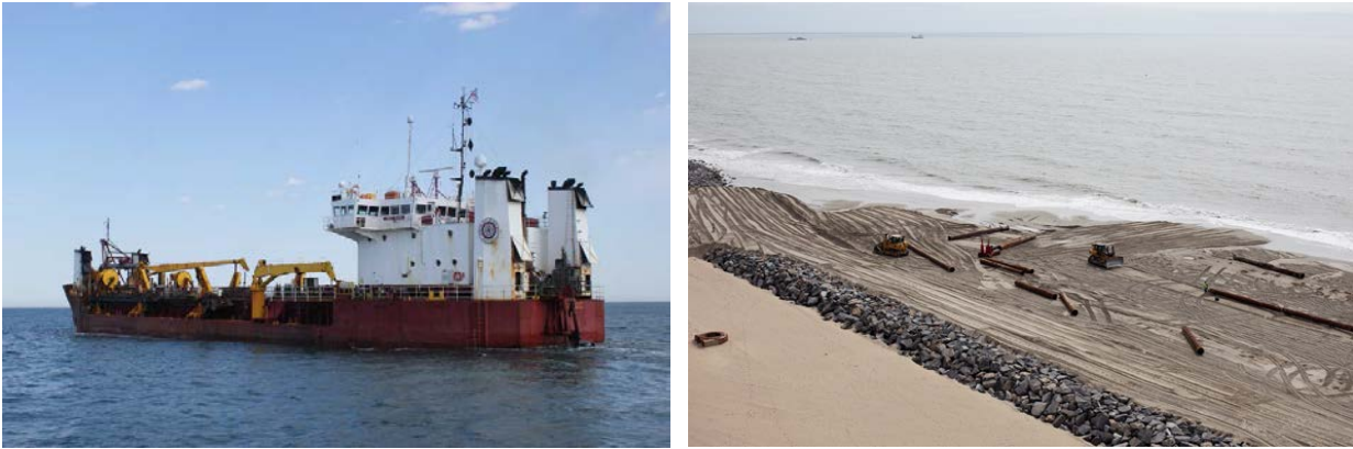
Figure 2.3-3. Dredging and Sand Placement Process, Trailing Suction Hopper (left) and Bulldozers Grading Discharge Sand (right)
